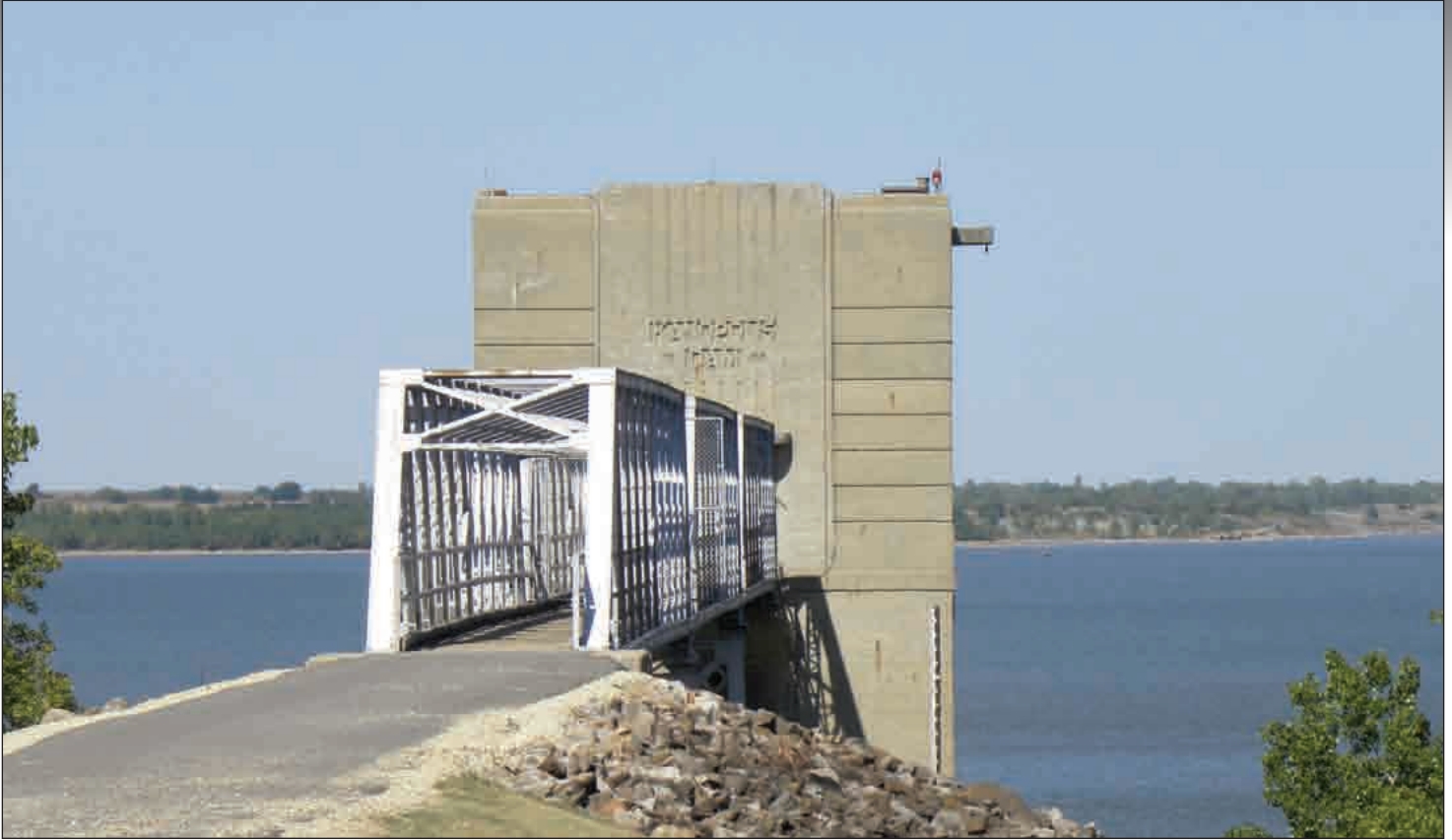
The control tower at the south end of Kanopolis Reservoir Dam, was built in 1948 and houses the heavy mechanisms that operate the gates that control water releases. For security reasons, no photos of the interior of the tower are allowed.
